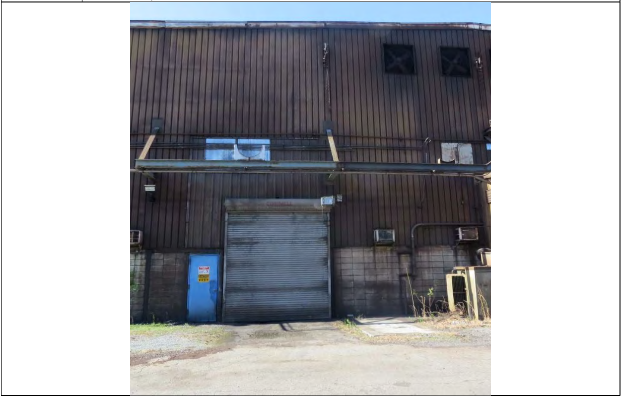
PHOTO 2 Location: North Wall of Bay 2 Description: Duct Supports Penetrating Siding
